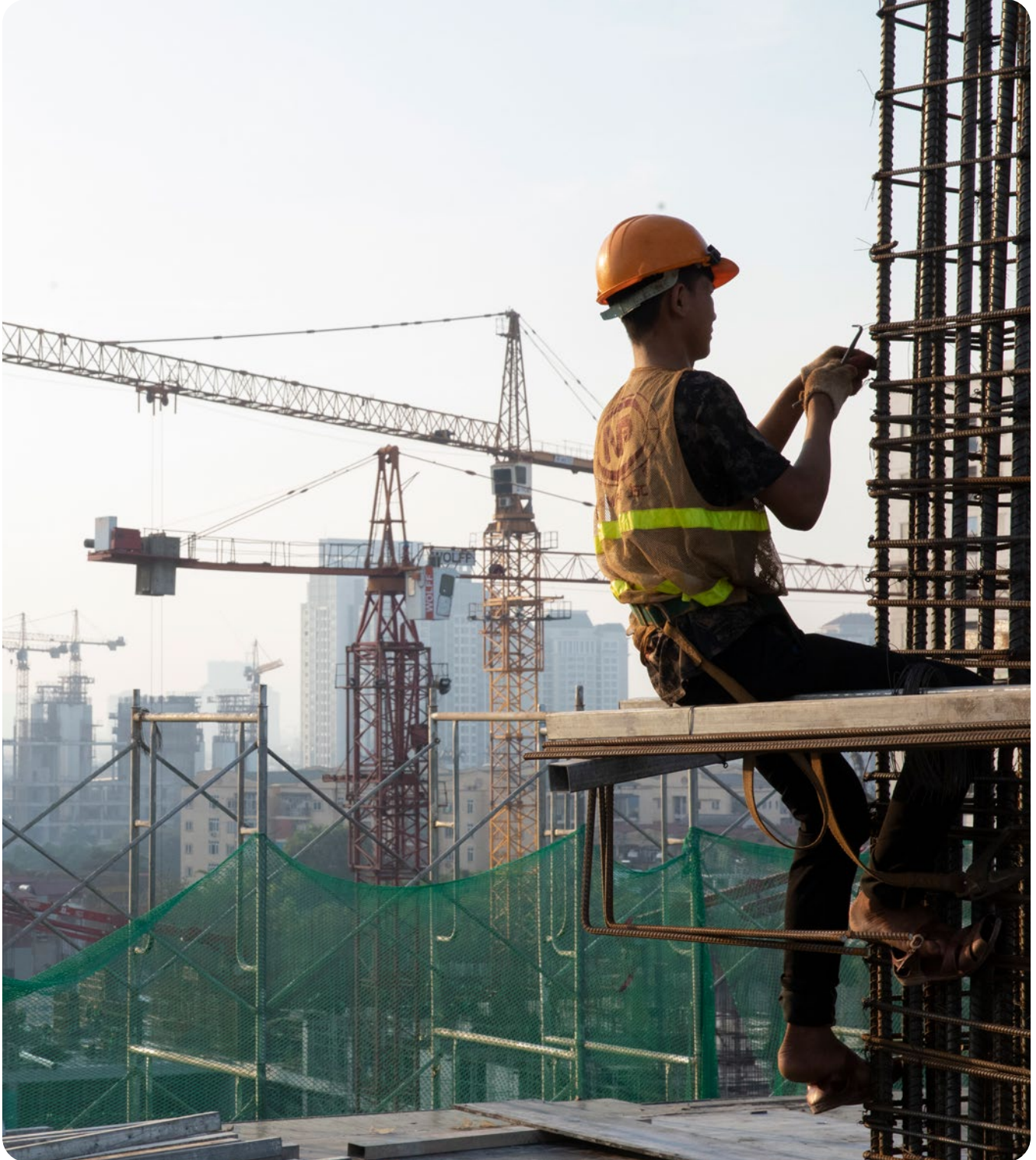
Construction worker preparing to pour concrete on an upper floor of the EcoHome apartment complex in Hanoi, Viet Nam. The finished towers will be EDGE certified and provide 2,197 affordable green apartments. Photo: © Dominic Chavez/IFC
